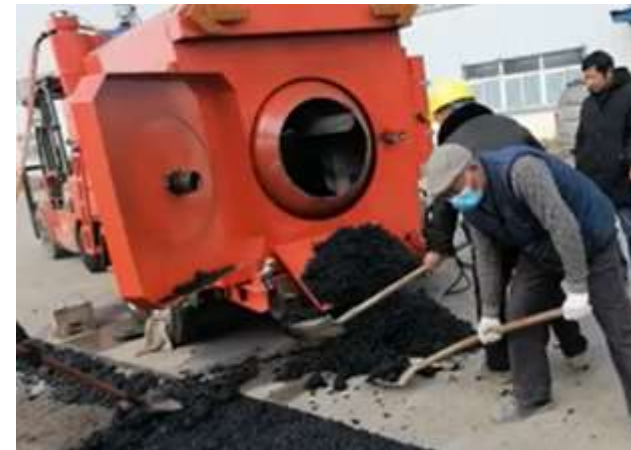
PORTABLE HEATING EQUIPMENT FOR CAPM FOR PATCHING
