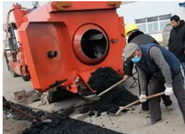
Portable Heating Equipment for CAPM for PATCHING.
